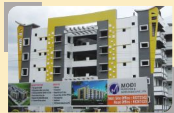
Main Road View
