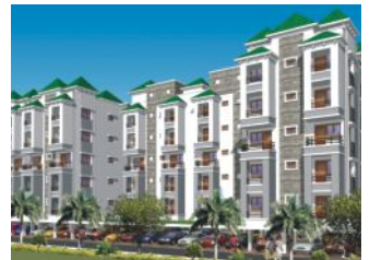
GREENWOOD RESIDENCY Kowkur, Bolarum, Secunderabad 345 flats on 6 acres of land
